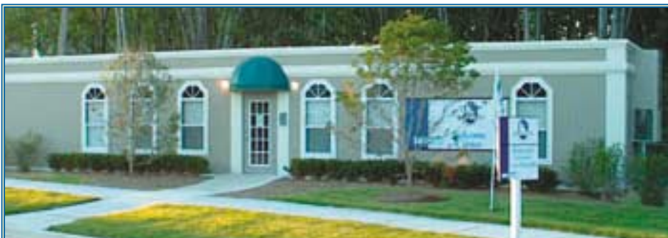
Sales are strong for temporary offices with higher ceilings and upscale finishing.
